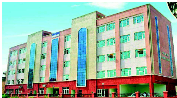
GPOA Building Jalandhar
