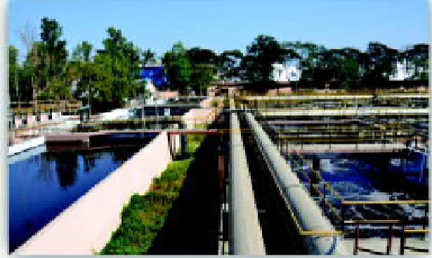
Upgradation & Augmentation of STP at Surat (Gujarat)
