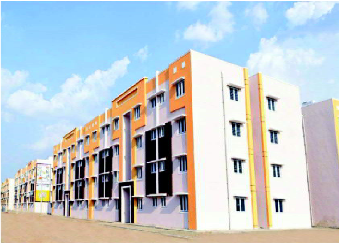
Houses constructed under AHP Project in Tamil Nadu
