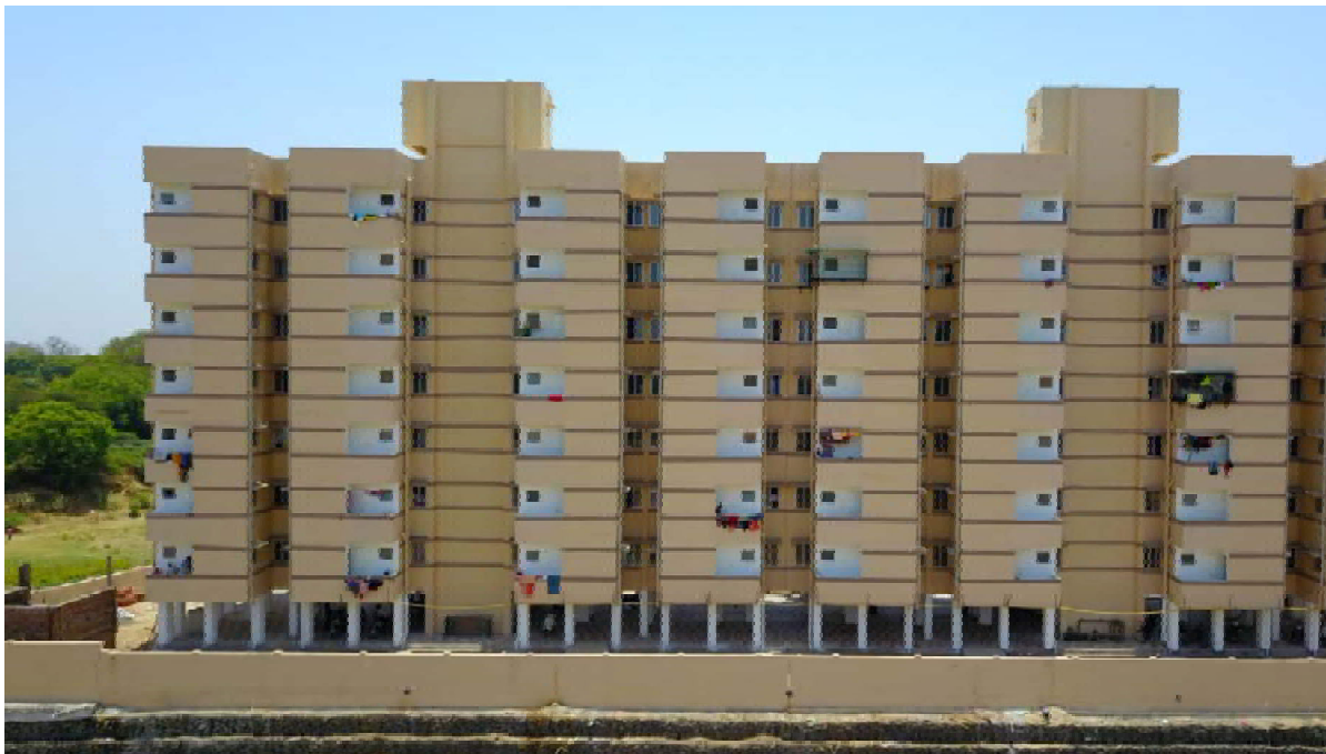
Construction of houses under ISSR in Gujarat
