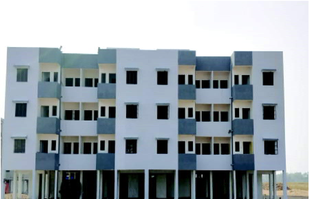
Houses constructed under AHP Project in Madhya Pradesh
