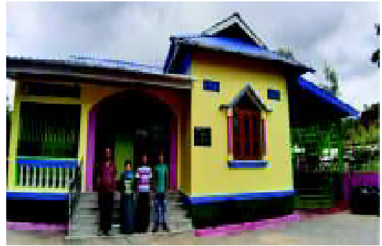
Houses constructed under BLC Project in Manipur
