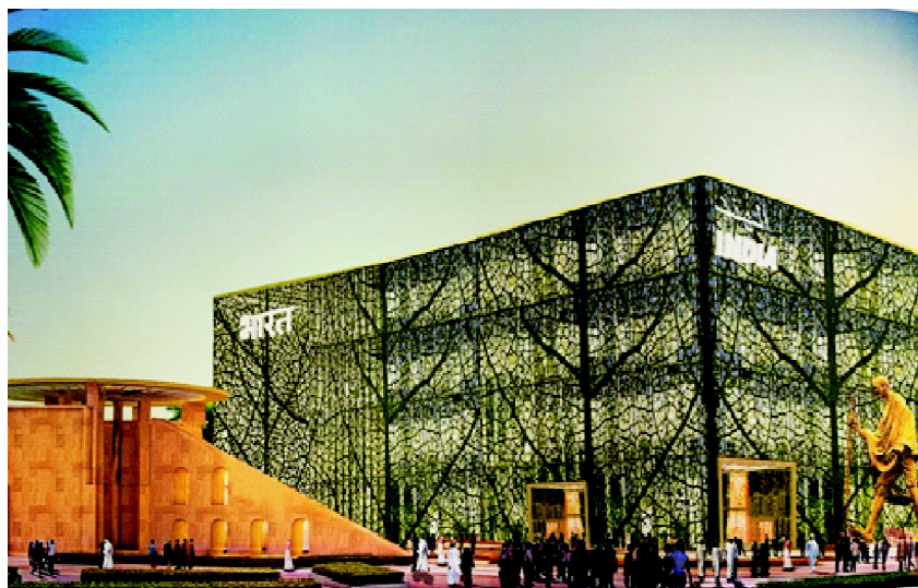
Construction of Indian Pavilion at Dubai World Expo, 2020
