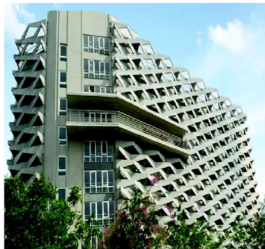
Screening of Utilities
