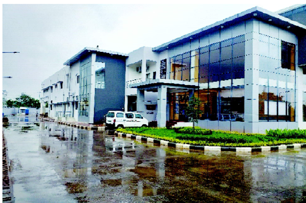
Figure 9: Kitchen Building - CSR Silvassa Project
