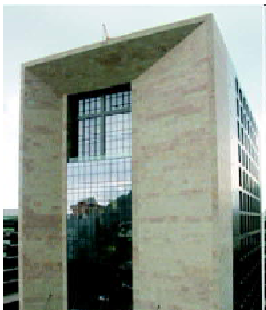
Construction of New Supreme Court Building, Port Louis, Mauritius
