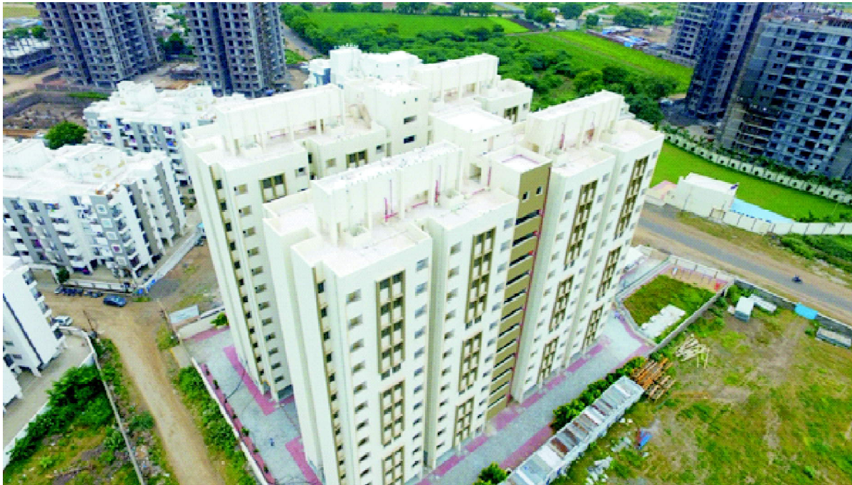
Houses constructed under AHP Project in Gujarat
