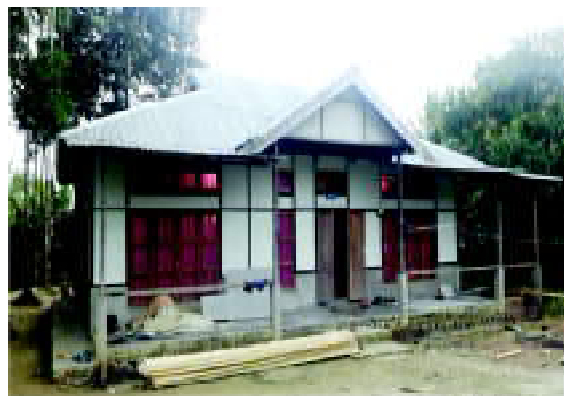
Figure 1: Lower Income Group (LIG) housing unit at Chakma Autonomous District Council, Mizoram
