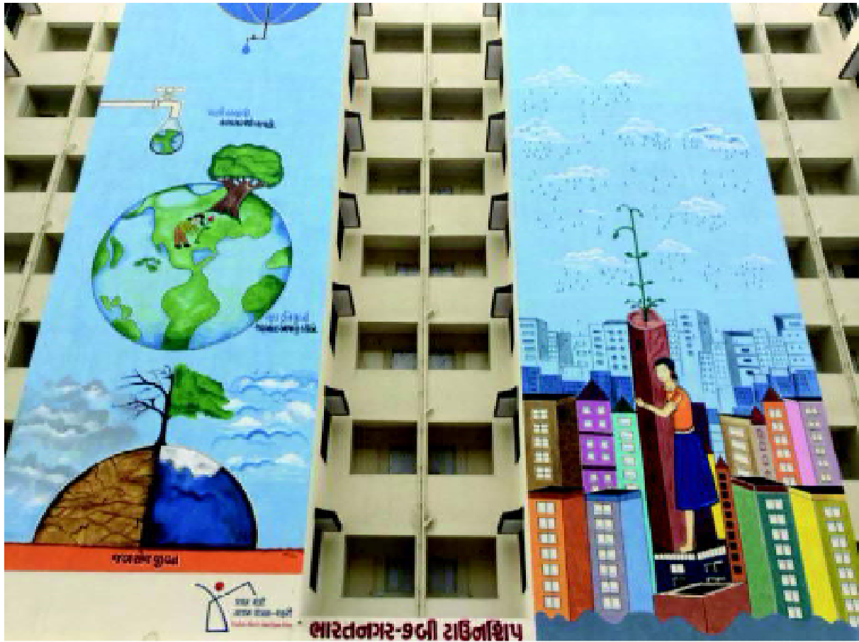
Construction of houses under ISSR in Gujarat
