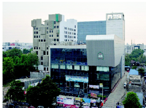
Figure 4 : APMC Building , Surat, Gujarat
