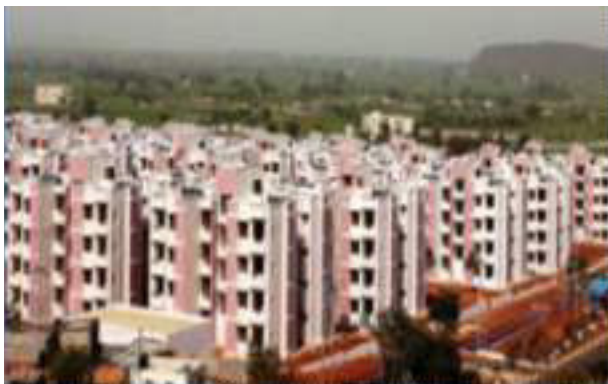
CRPF Jawan Barracks and Housing Colony, Gwalior, Madhya Pradesh
