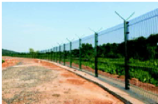
Fencing work, Meghalaya
