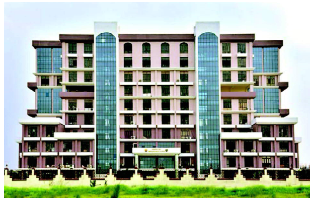
Administrative Building for BSF South Frontier, Kolkata
